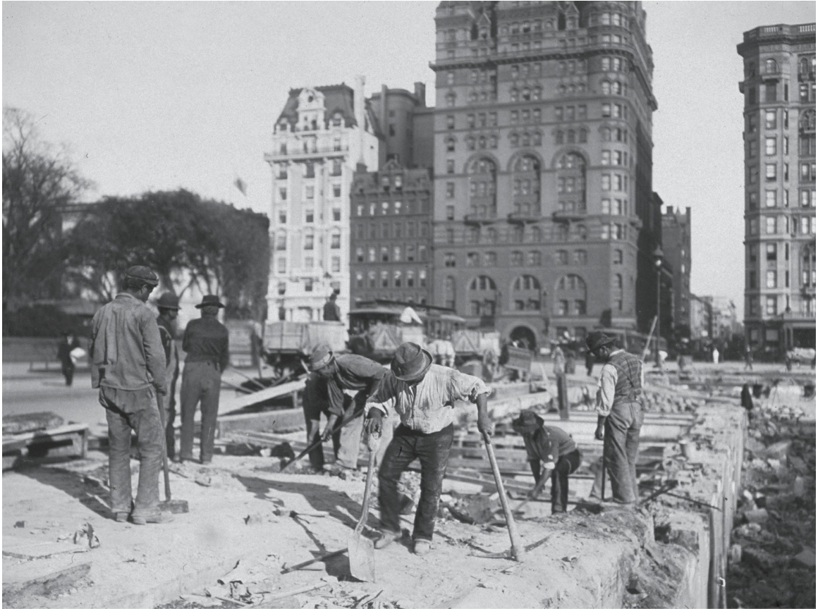
DEMOLITION: A dozen years after opening, the first Plaza was torn down in the space of just eight weeks. In its place, a new white marble edifice, which still stands today, began rising. Here, workers in 1905 remove the foundation of the original Plaza. Photo by Museum of the City of New York / Byron Collection / Getty Images
