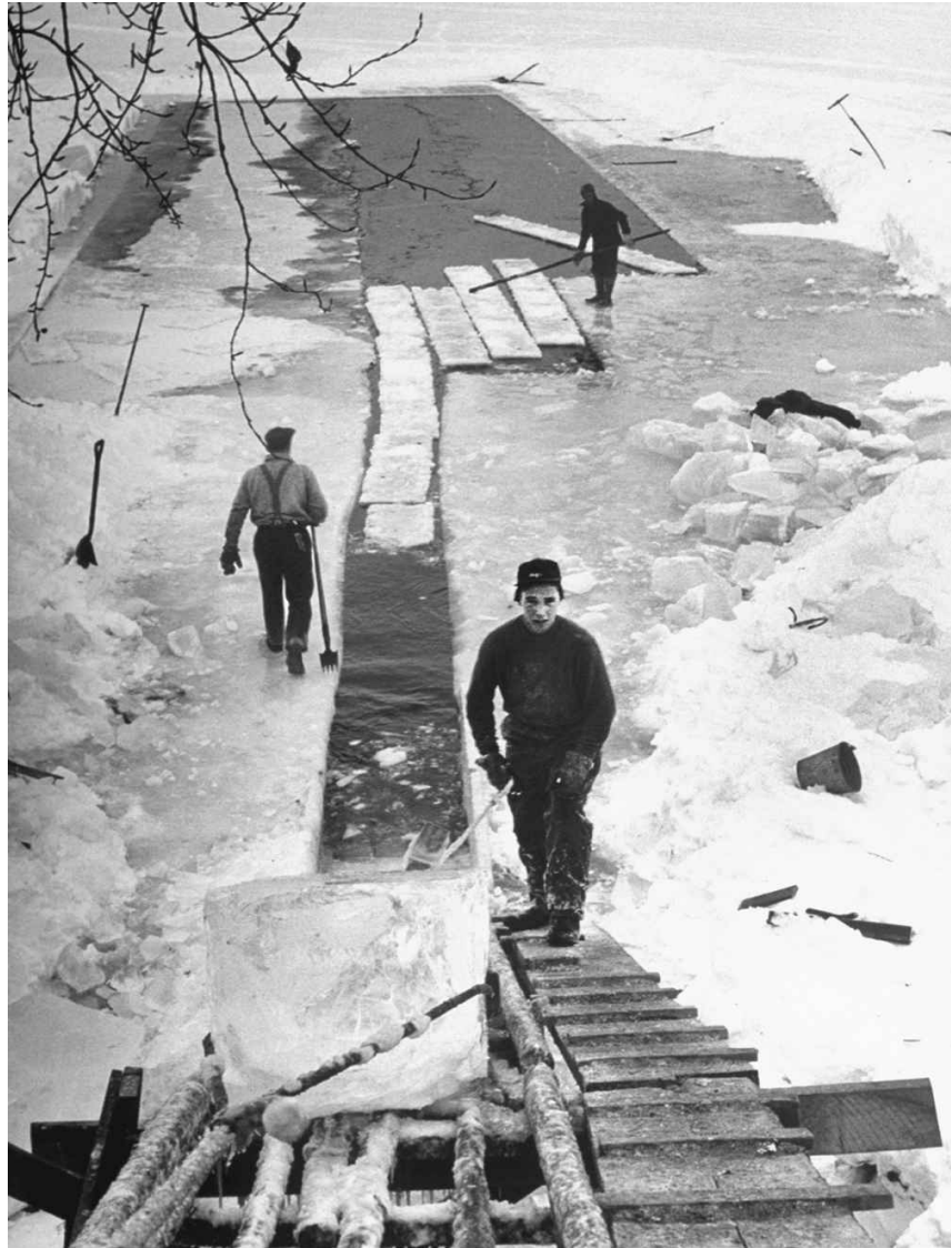
Ice blocks being cut from a lake are floated in water, then up a runway to a storage house, 1950.
