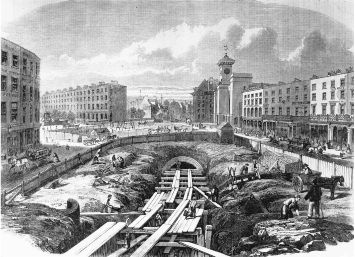
Workmen make progress on the Metropolitan Line underground railway works at King's Cross, London.
